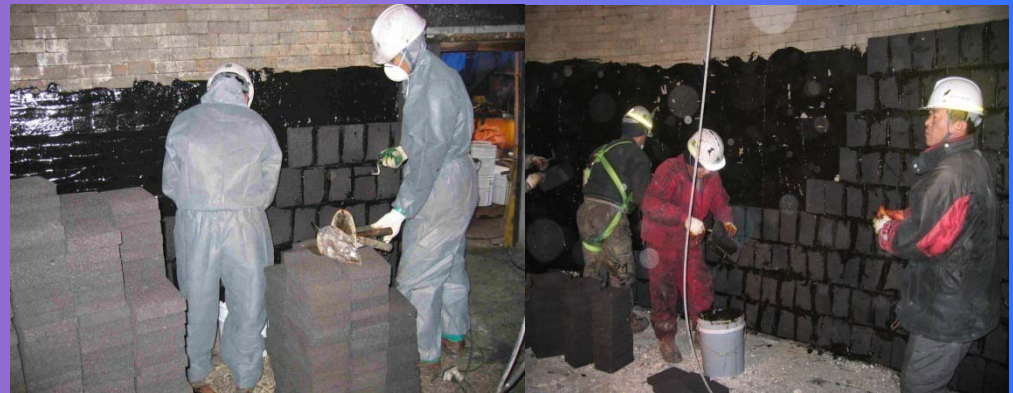
Glass Block working (GI-180)
