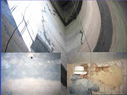
Surface Repair (Epoxy Mortar;GInsulation-183)
